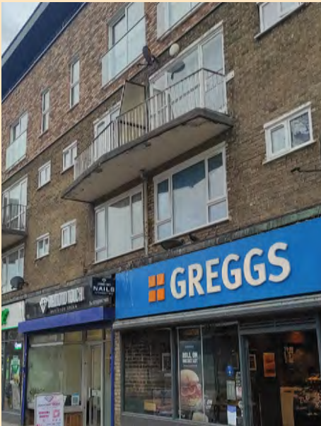
Expressive balconies, Hemel Hempstead New Town
