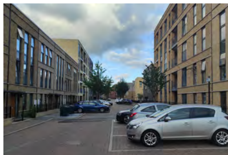
Parking incorporated into the public realm in a way that means the spaces could be reclaimed for a different use in future.
