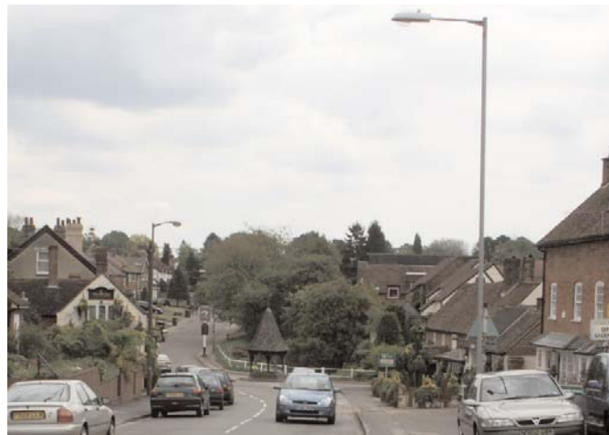
The streetlighting in the High Street is a continuation of the highway lighting on Chipperfield Road.
