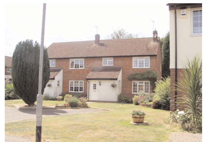
4. Semi detached house with on-street parking, communal front garden and private rear garden Hempstead Road.
