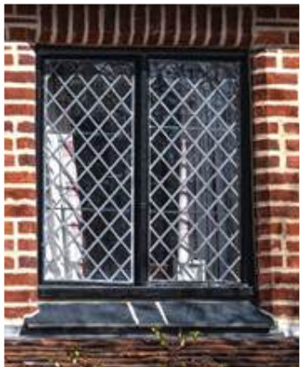
Window at No 41
