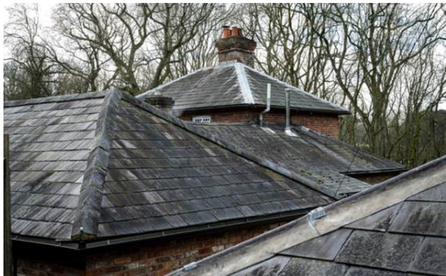
Home Farm slate roofscape
