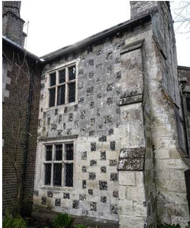
Wall at Manor House: Flint and Totternhoe Stone
