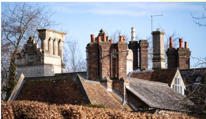
Roofscape of chimneys at the Manor House
