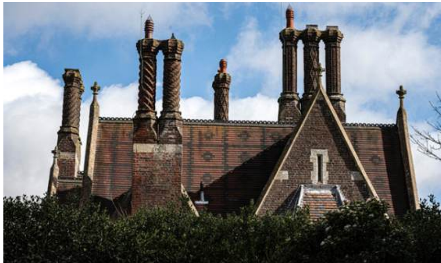
Little Gaddesden House – decorative chimneys and tile pattern
