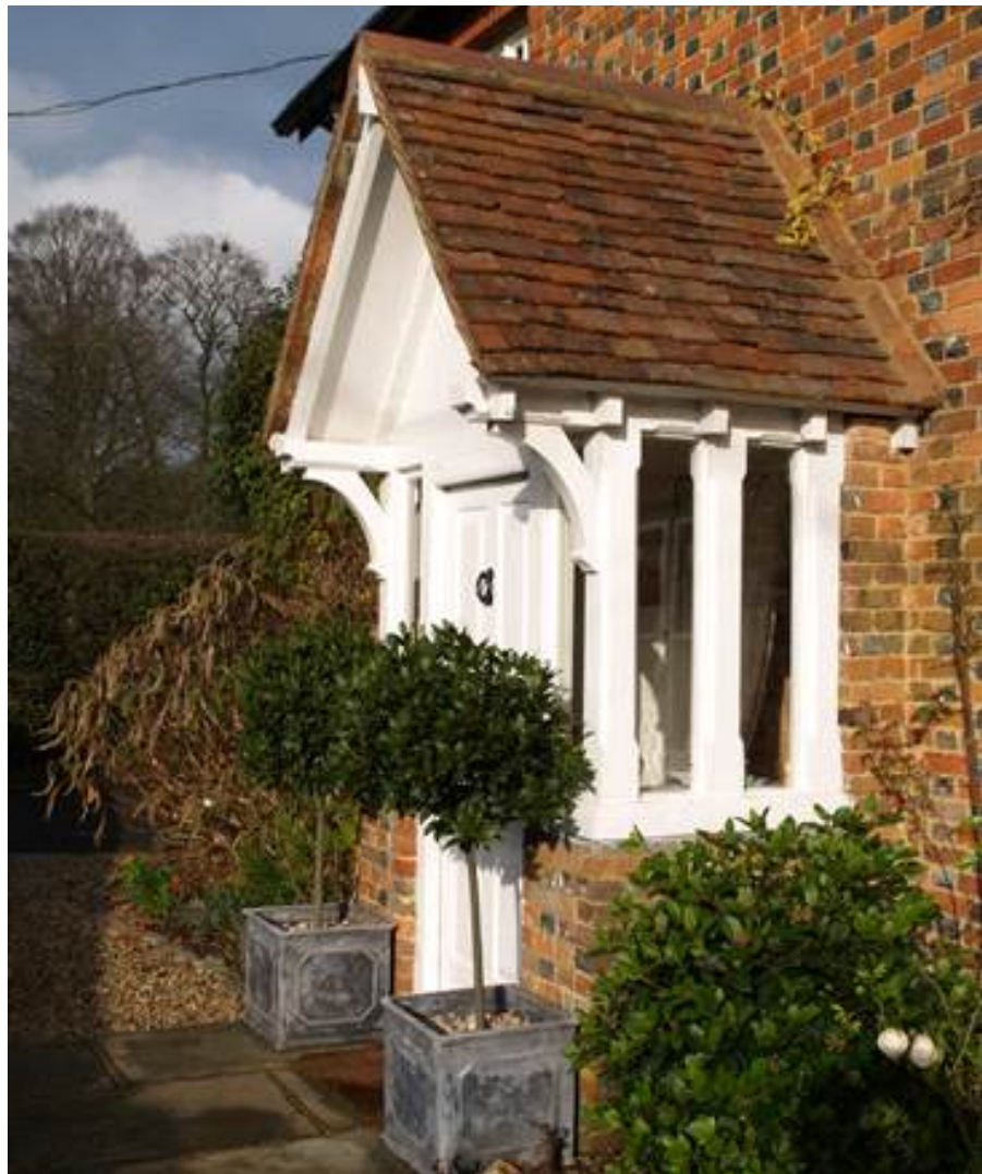
Porch at Keepers Cottage
