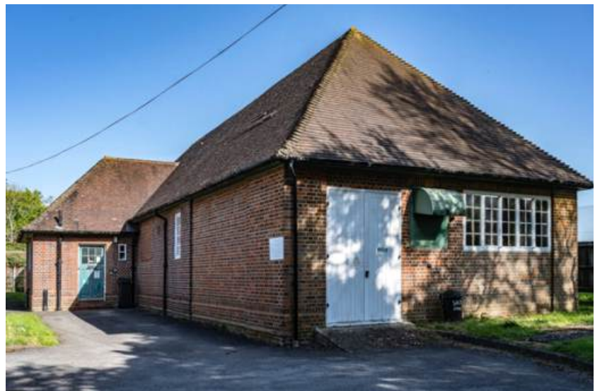
Telephone Exchange building
