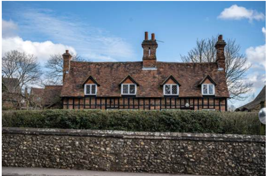
No 22/23: Timber-framing, infill brickwork, peg tiles and leaded light casement windows. Front boundary flint wall and hedging.
